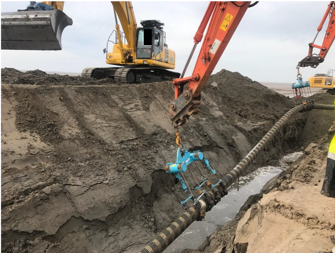
Plate 4.5 Cable being placed in an excavated trench (Walney Extension Offshore Wind Farm)
