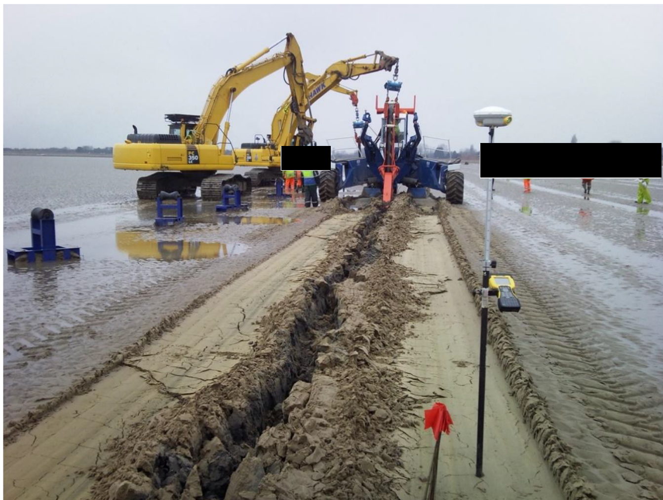
Plate 4.6 Cable being buried using a plough with excavators (Thanet Offshore Wind Farm)
